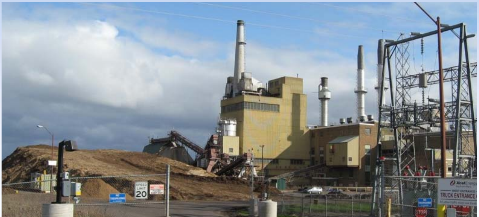
Xcel Energy's Bay Front Plant sits along the Chequamegon Bay of Lake Superior in Ashland, WI. The 73MW plant is phasing out its use of coal. In 2007, 206,000 tons of wood was burned at the plant.
