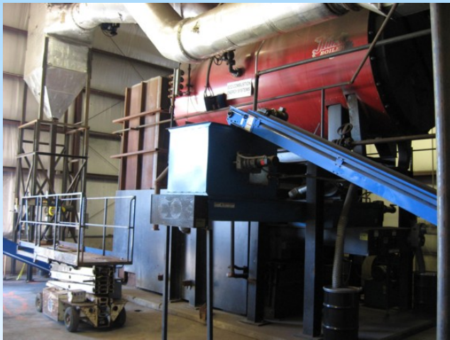
(clockwise from bottom left) Outside the building that houses the burning of the manure, the bag house works as a filter to take out particulate so it is not released into the atmosphere. The ash can then be used as concentrated fertilizer that is odor free and easy to haul. / The boiler and bio-mass burner. 2000 dry tons of manure per hour is burned at 2000 degrees Fahrenheit./ The control room shows how the process is working and at what capacity the system is operating. / The conveyor which takes the dried manure to the hopper where it is then put into the combustor.
